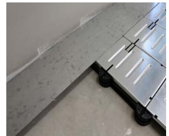
Galvanized Steel Filler Plate to be Cut-to-Fit at Perimeter Walls
